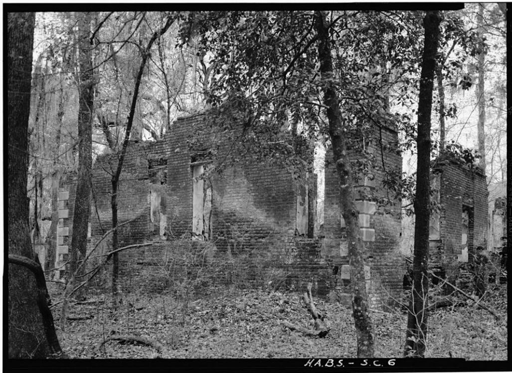
Figure 2. Crowfield Hall Ruins, 1940 (HABS 1940).
